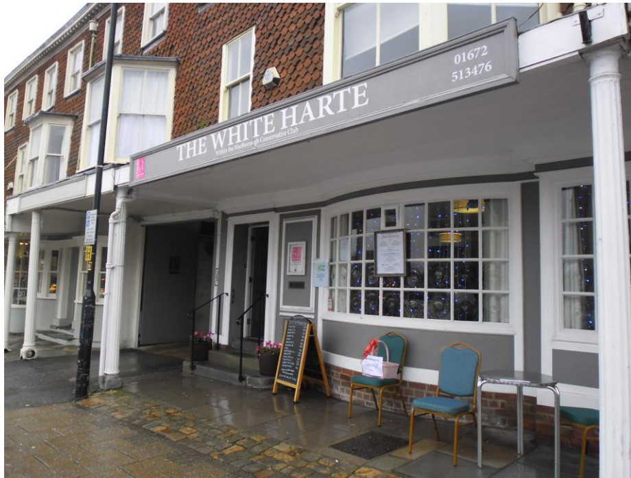
View of the principal elevation of the site
