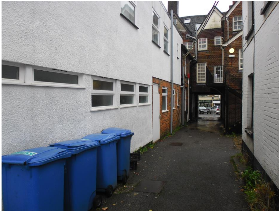
View showing the 1960s extensions to the rear of the site
